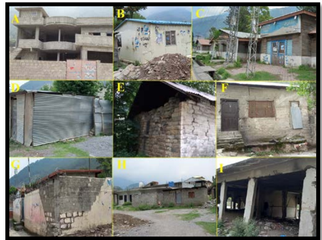
Fig. 2. (A) Adobe column and cement block wall proper columns and RCC/BCC lintel, (B) Pitched sloping with prefabricated sheets, (C) Wooden wall and roof with sheet, (D) Simple sheets, (E and F) No column or beams, (G and H) Hairline cracks and plaster damages, broken, Seepage, and (I) Destroyed shops on October 8 th , 2005 Earthquake at Pakistan.
