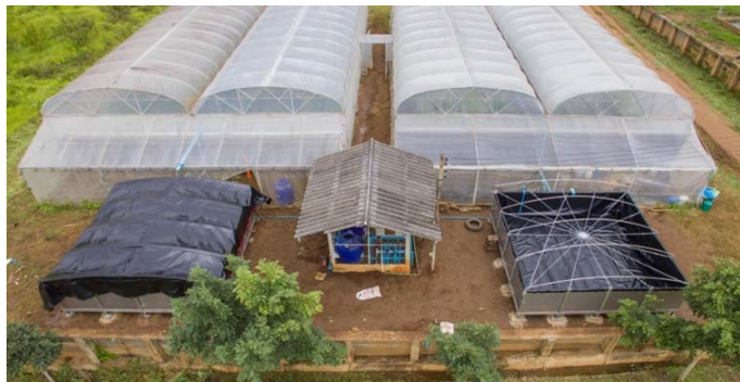
Fig. 9. Two prototypes of the developed reservoir with a capacity of 27,000 liters each installed at greenhouses at the Royal Agricultural Station Pangda.
