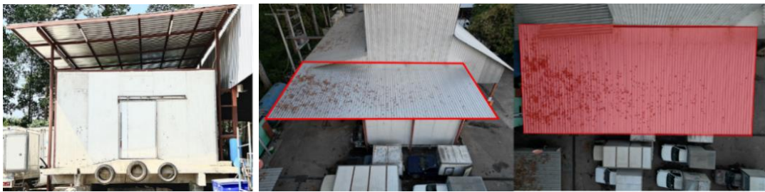
Figure 1 Cold storage room and PV rooftop area
